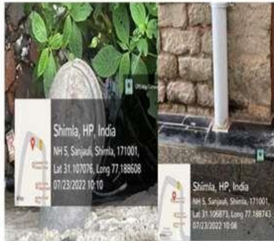
PVC pipes used to reach the rain water to the tank from various buildings' roof
