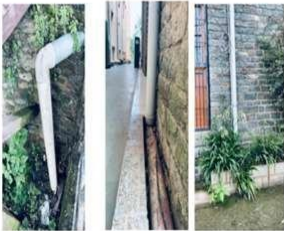
PVC pipes used to reach the rain water to the tank from various buildings' roof
