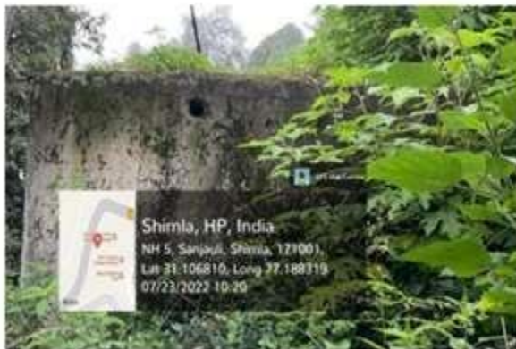
Rain Water Harvesting Tank
