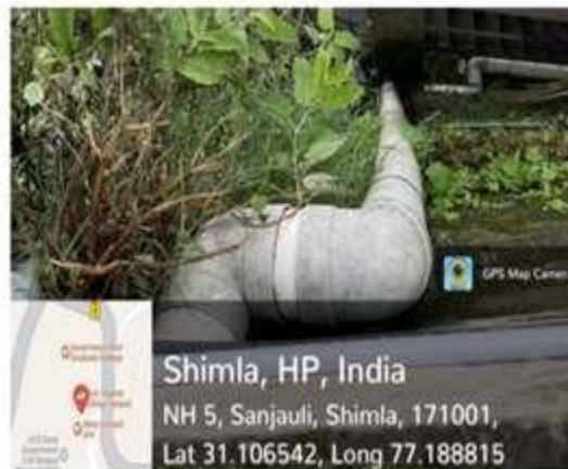
PVC pipes used to reach the rain water to the tank from various buildings' roof
